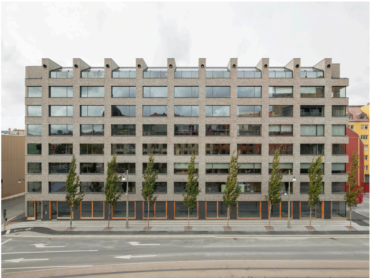
Figure 19. Facade with newly manufactured bricks (Olsson Lyckefors, n.d)
