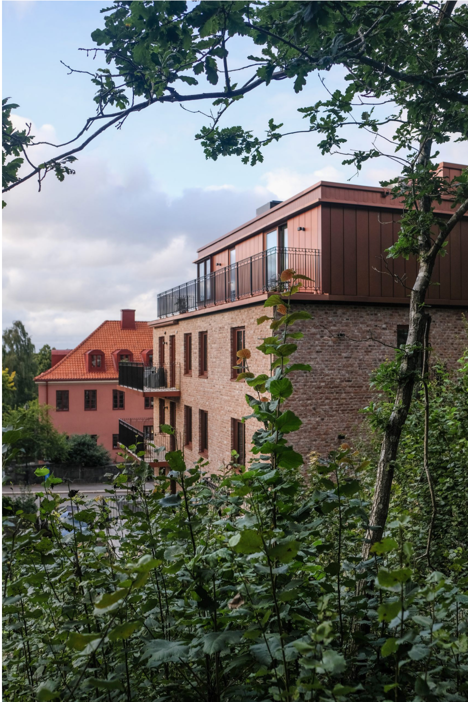
Figure 7. Facade from Villa Lorensberg. (Inobi, n.d)
