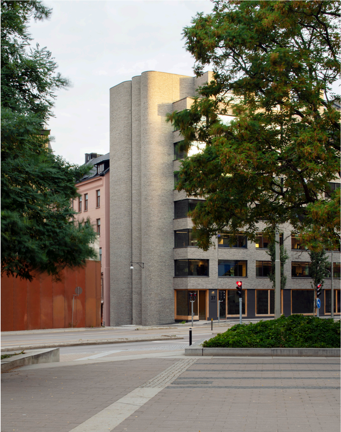
Figure 18. Facade with newly manufactured bricks (Olsson Lyckefors, n.d)
