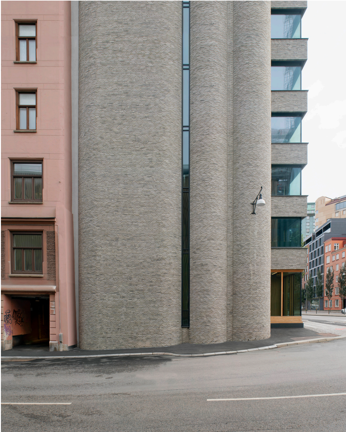
Figure 20. Facade with newly manufactured bricks (Olsson Lyckefors, n.d)
