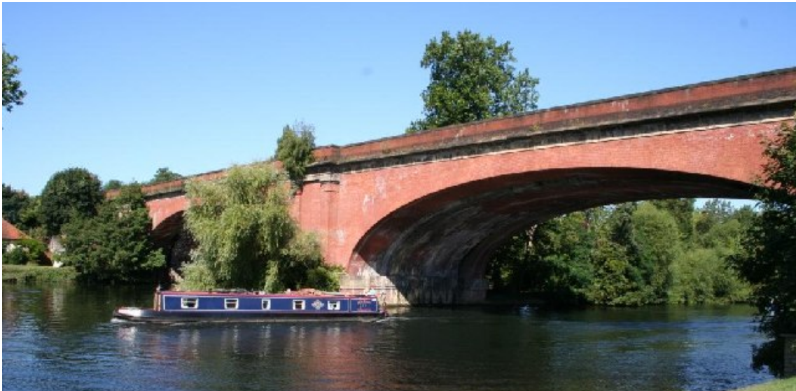
Figure 1.1: Maidenhead Railway Bridge designed and constructed by Isambard Kingdom Brunel. Photo by Stephen Daghish licensed under CC BY-SA2.0
