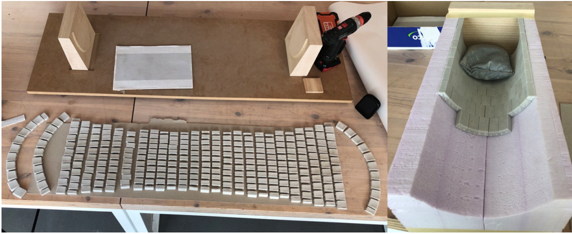
Figure 4.4: Left: All the blocks sorted according to the numbering system. Right: Assembly process in the formwork
