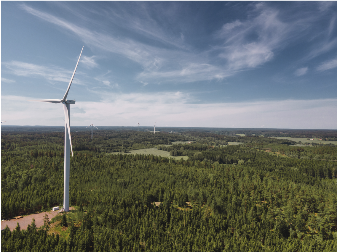
Figure 2.2: SR Energy's wind park Örbacken [11].
