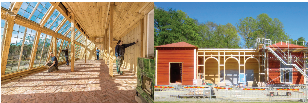
Phase 4. Greenhouse, interior and constructure of The orangery (pictures from gunnebo.se)
