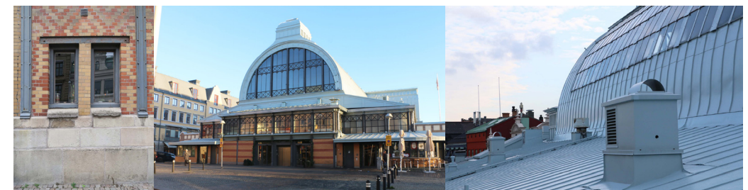
Fig. 20. Original narrow windows from 1906 Source: Tyréns AB (2019)
