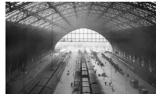
Fig. 5. St. Pancras Station, London, 1895 Source: Historic England / Media Storehouse
