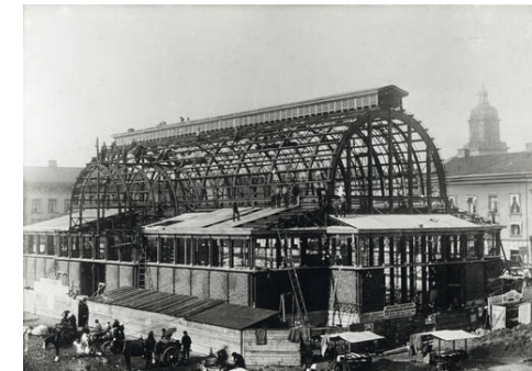
Fig. 9. Stora Saluhallen under construction (1888) Source: GSM / Tyréns AB (2019)
