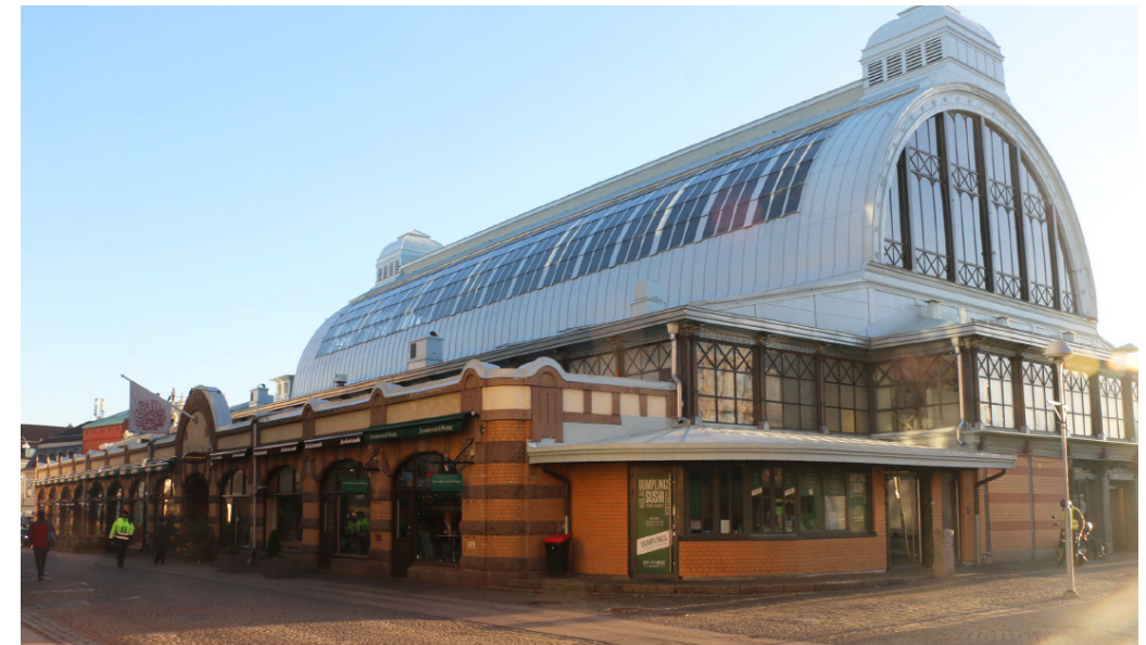
Fig. 16. North/West facade, 2018. Cast-iron windows and skylights allow natural light into the main hall. Source: Tyréns AB (2019)
