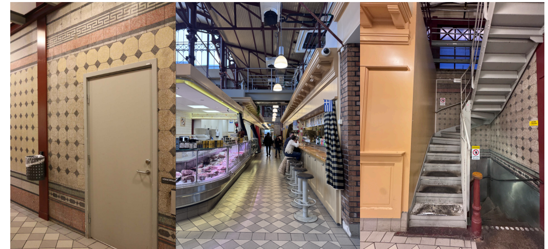
Fig. 26. Original terrazzo tiles along the western wall. To the left, a later addition with a simpler pattern but matching colors. Source: Tyréns AB (2019)
