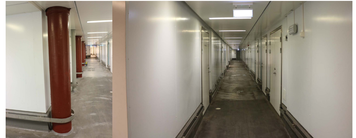
Fig. 32. Original 1888 cast-iron columns in the basement corridor. Source: Tyréns AB (2019)
