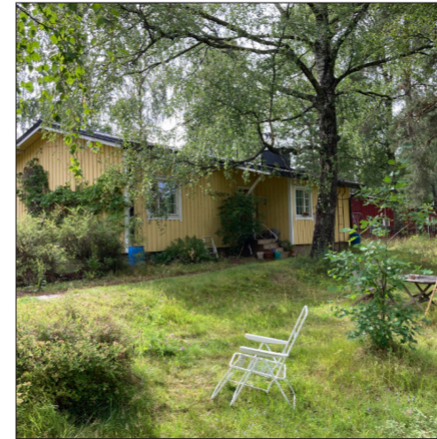
Neighboring building to the northwest.
