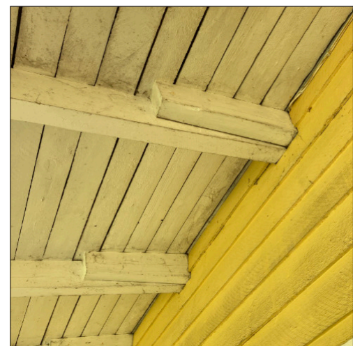
When the house got an expansion somewhere between 1962 and 1992 the existing roof beams simply got extended.
