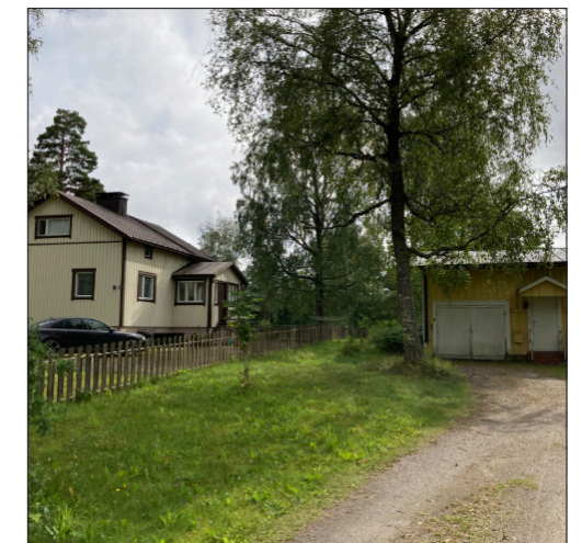
Neighboring building to the southeast.
