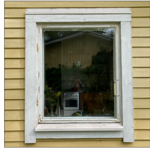
All windows are of a traditional double glass type where the exterior frame opens outwards and the interior one opens to the interior. There is a metal sill above and under the window.
