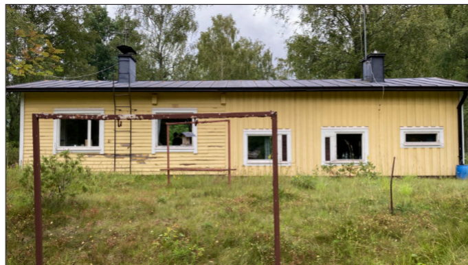
Facade to the southwest.
