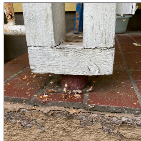
The columns holding up the roof above the entrance is raised from the foundation by a metal footing.
