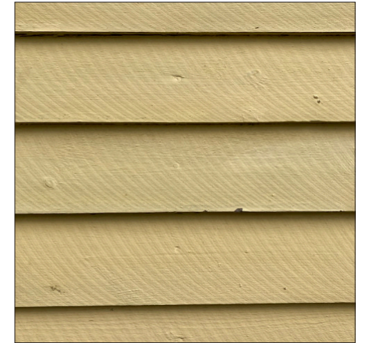
Feather edge timber cladding with visible marks from circular saw during production was used on the original building. Under the yellow acrylate paint there is signs that the facade use to be brown.
