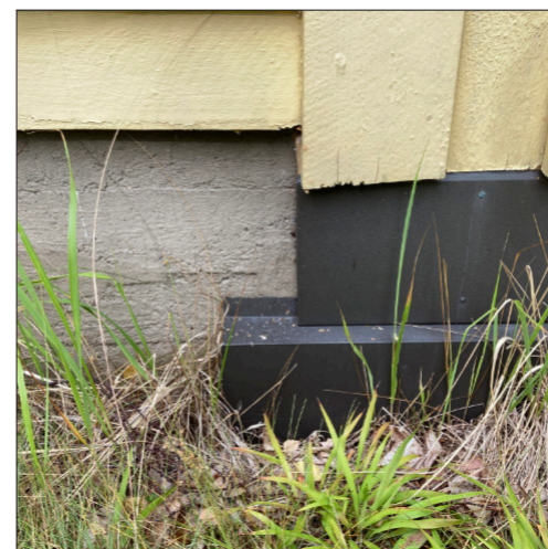
Parts of the foundation have been covered in sheet metal to create a barrier to the ground at parts where the building turns to a souterrain type, no one knows what can be found behind it.
