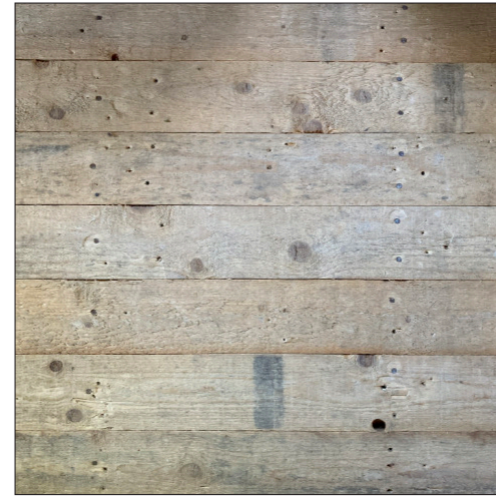
95mm wide raw cut timber floorboards were found under linoleum carpet. Underneath there is sawdust used as insulation.
