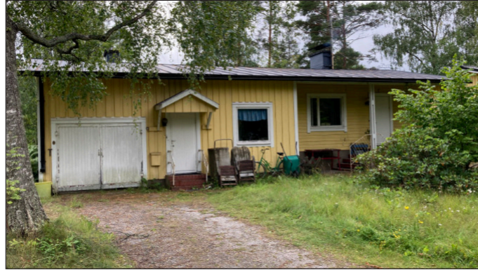
Facade to the northeast.
