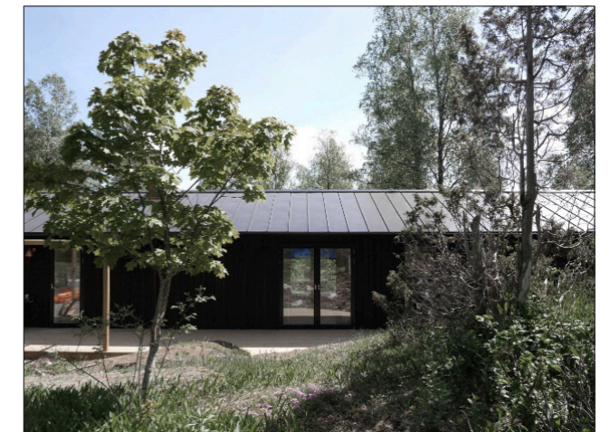
Not much of the original cabin is left to be seen in the final building. The transformation can be seen as one from cabin to a contemporary building style where the timber of the facade and the metal sheeting of the roofing are in a uniform tone of color. Double glass doors are place to match the intended interior program and plan.
