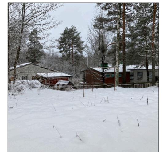
Neighboring building to the southwest.
