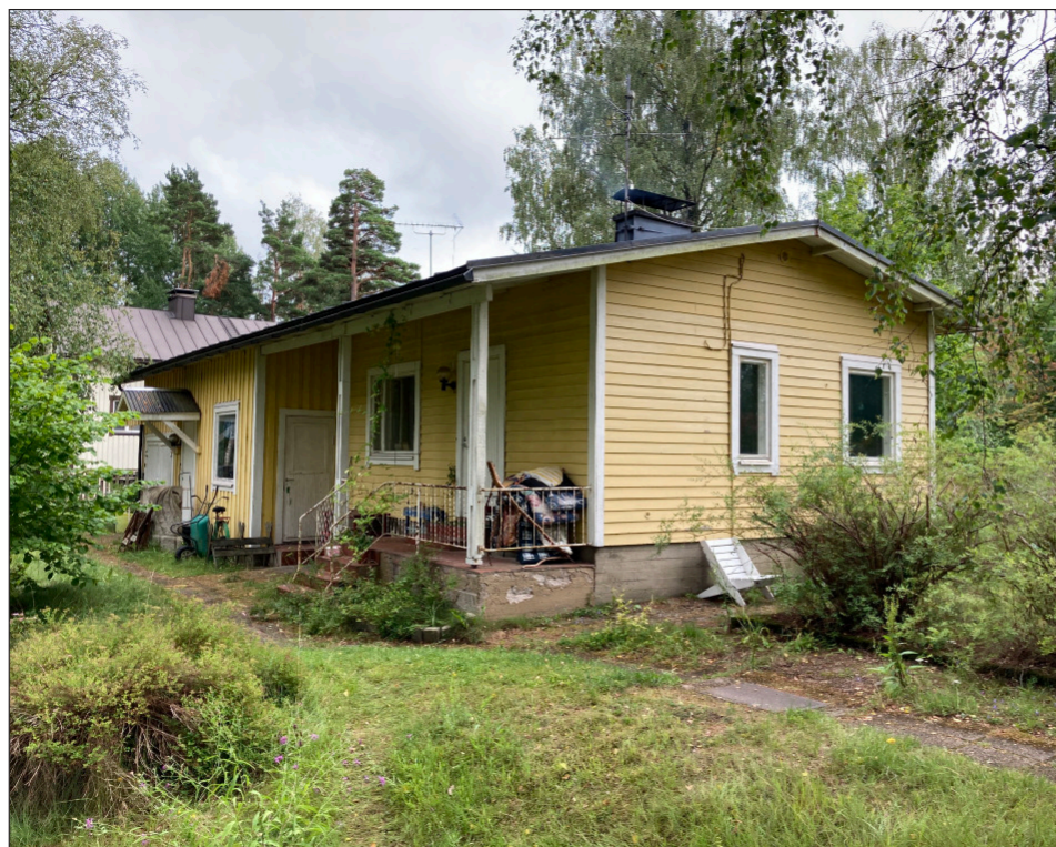
Existing building, view from northwest.
