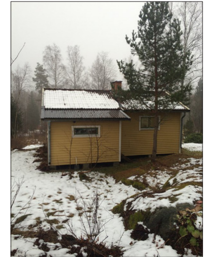
The original cabin and the surrounding landscape is ultimately a starting point for inspiration but also a boundary or restriction for the building project. What would you save? Change? Reuse? Rebuild? It really is an interesting starting point compared to a clear plate.
