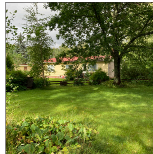
Neighboring building to the north.
