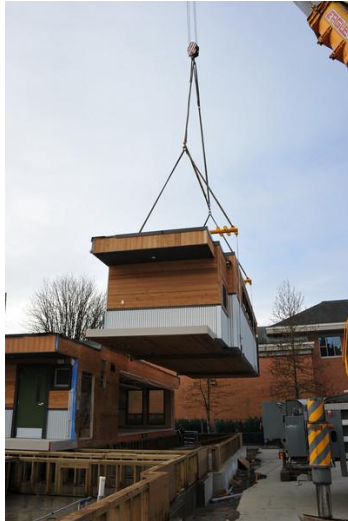
Figure 8 An example of 3D-volumetric modules. These modules have floors, ceilings and four walls prefabricated. Retrieved from Province of British Columbia (2011).
