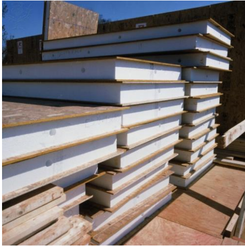
Figure 7 An example of 2D-panels, specifically, timber panels with foam insulator. Retrieved from Britannica ImageQuest (n.d.b).
