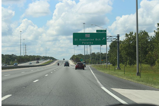
Figure 1.1: Highway exit in Florida, where the right lane marker, if continuing straight ahead, is not following the lane of interest. Photo: [1], CC BY-SA 4.0
