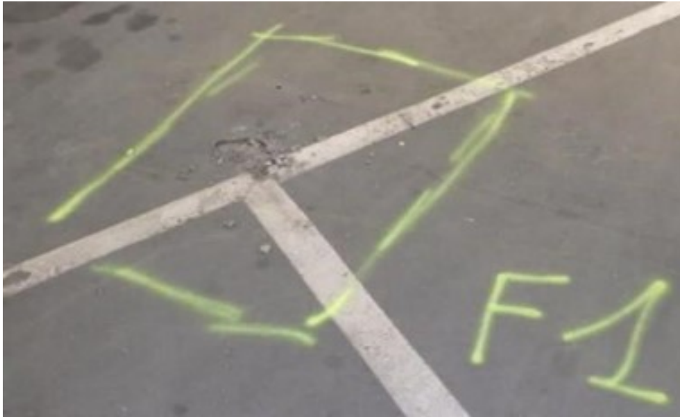
Figure 3.6: Location of window F1 in the second floor from Afry reports.
