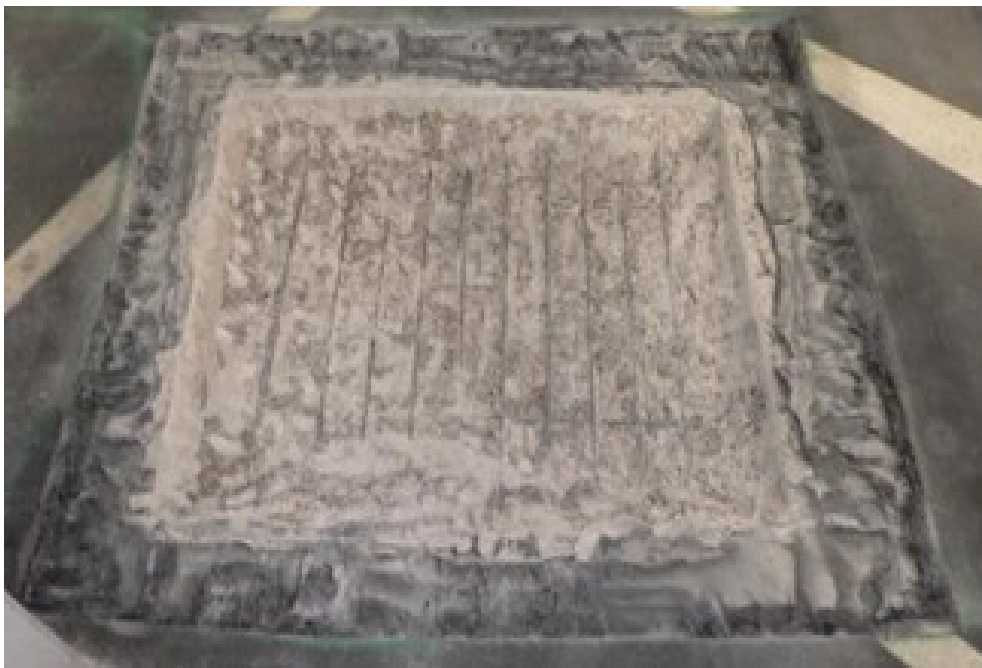
Figure 3.4: Reinforcement status in window F3 from Afry reports.
