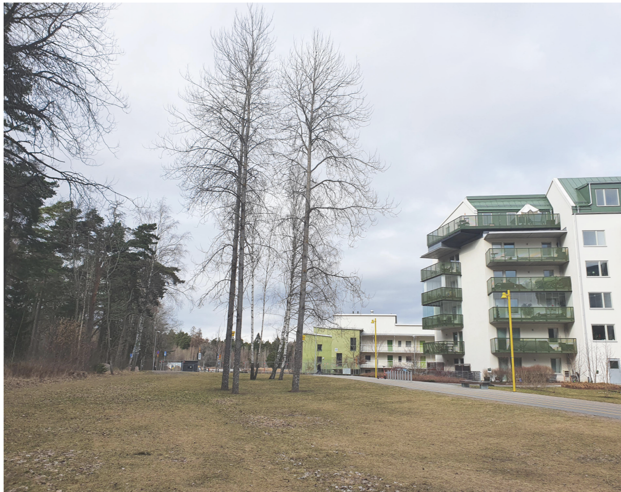
The site viewed from south
