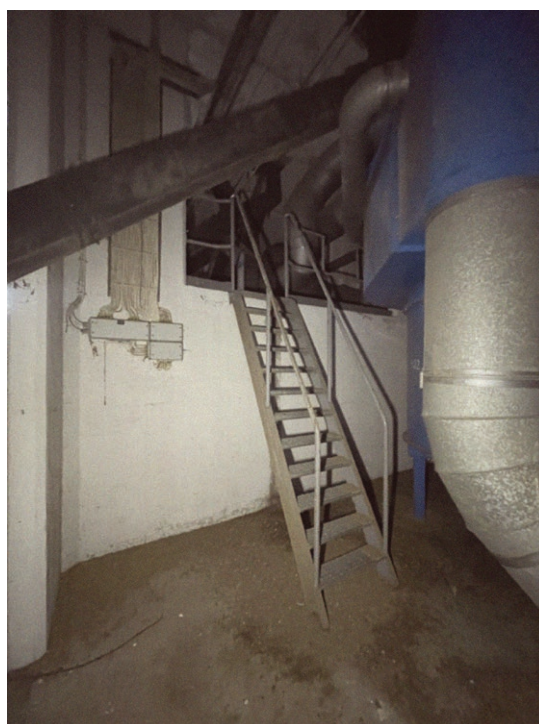
Figure 37. Interior photograph, mezzanine.
