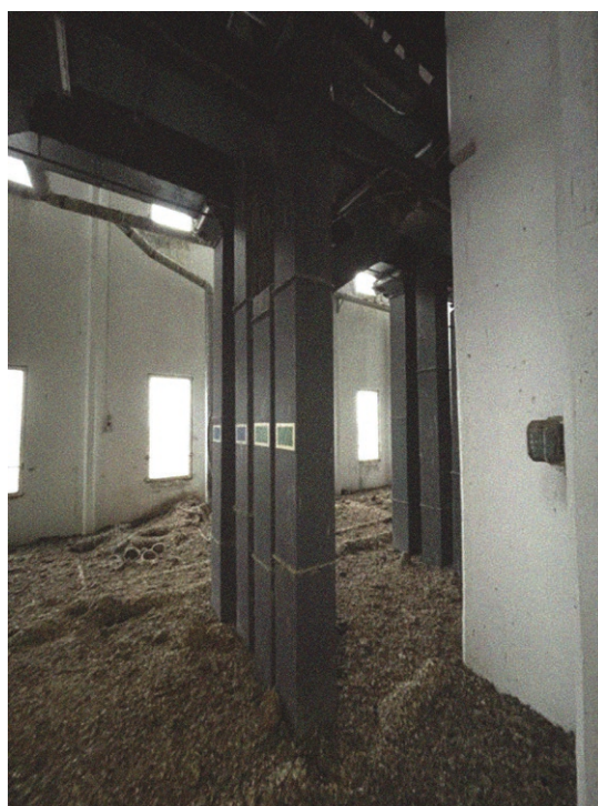
Figure 41. Interior photograph, existing light intake.
