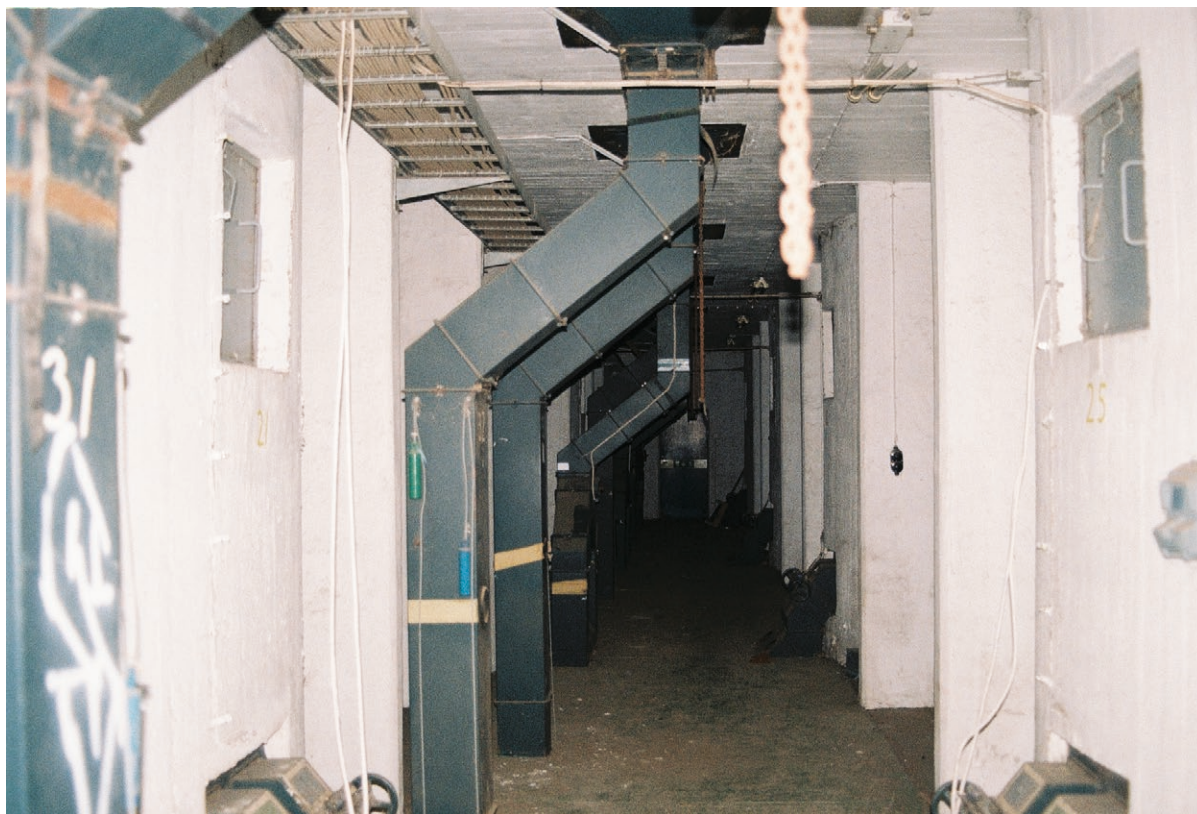
Figure 39. Interior photograph, center corridor.
