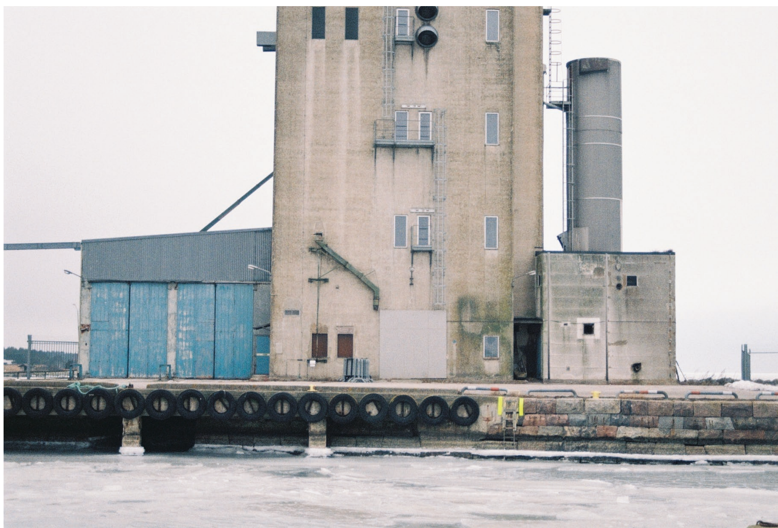
Figure 25. View on west facade.
