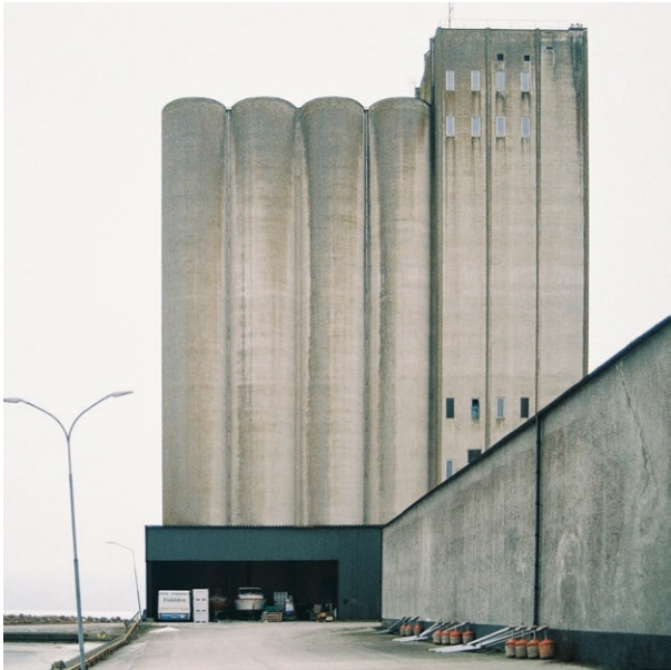
Figure 16. Existing view of new entrance.
