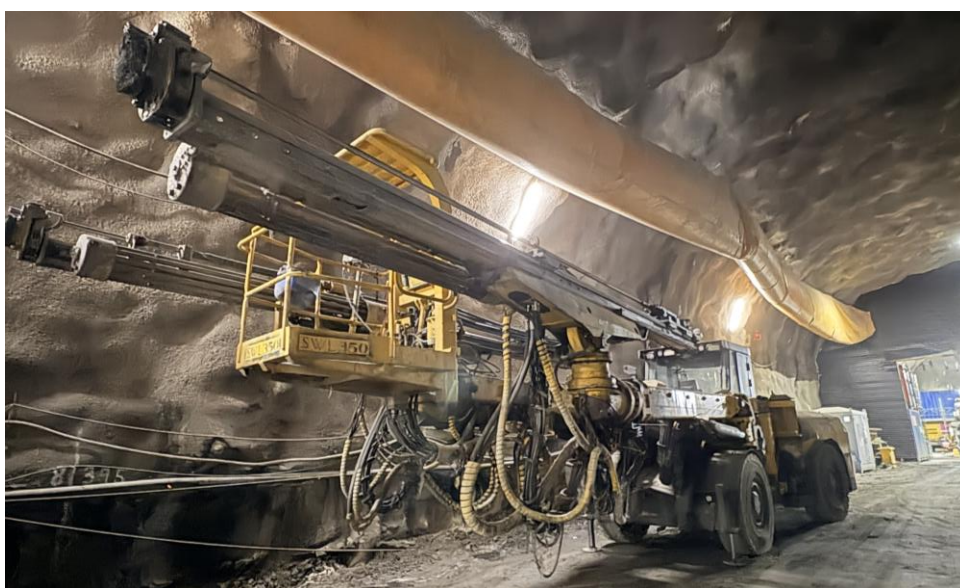
Figure 15 Bore Rig from the Service Tunnel, own image
