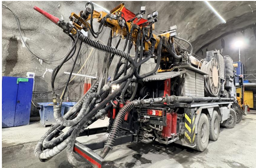
Figure 4 Shotcrete Machine, own image from the service tunnel
