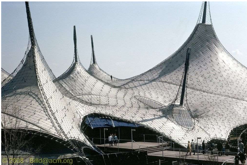
Figure 3.82 - Frei Otto's cable structure (Pinterest, 2008)
