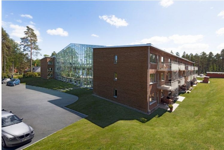
Figur 7. Boverian exteriört. (Boverian, 2015)
