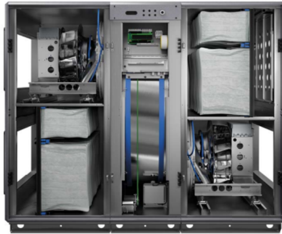
Figure 2.2: Overview of Swegon's air handling unit [9], reproduced with permission from Swegon
