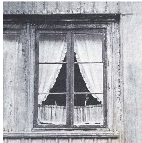
Figure 8. Close-up on the steel framed window in wooden façade.
