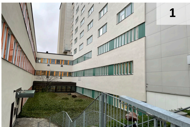
Courtyard between buildings in the north
