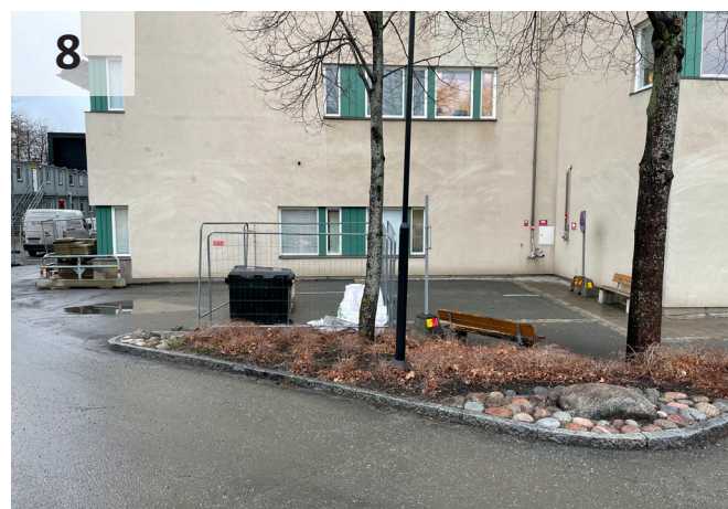
The corner of building 85
