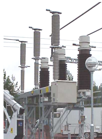
Figure 22 – Push BirkaNät Trial installation Nov 15 th 2000. Application: 132kV line/transformer protection. (from internal ABB PowerPoint presentation)
