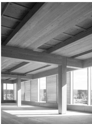
Fig 22. CLT & Glulam structures Wood Innovation Design Centre (© Michael Green Architecture)
