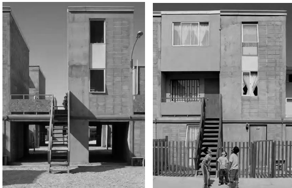
Fig 4. Quinta Monroy - initial house & five years later (© Elemental)
