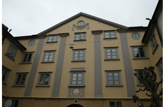
Figure left: Three floors are typical for Landshövdingehus. The ground floor in stone, and the two upper ones in wood.
