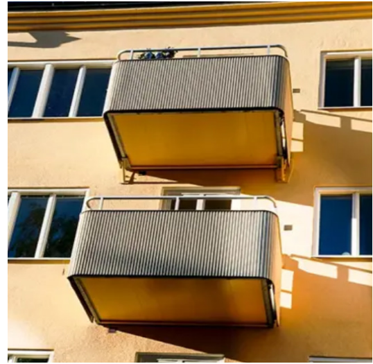
Figure 34: 'Sinusplåt' on balconies (Hogstad Aluminium AB, 2024)
