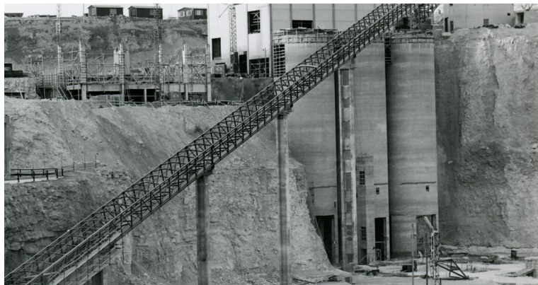
Figure 33. Silos and conveyor belt under construction (Skånska Cement AB, 1967).
