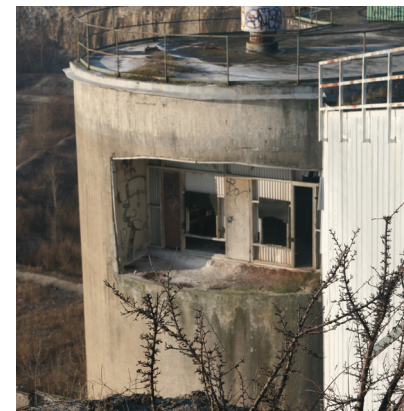
Figure 34. Existing opening towards east.
