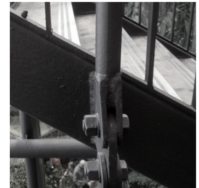
Figure 65. Tension rod detail.
