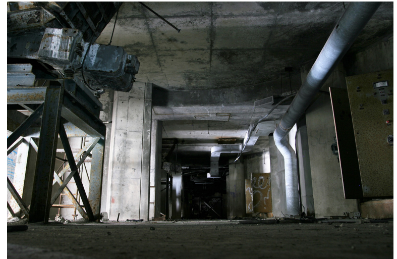
Figure 29. View of the 1st floor of the silos.
