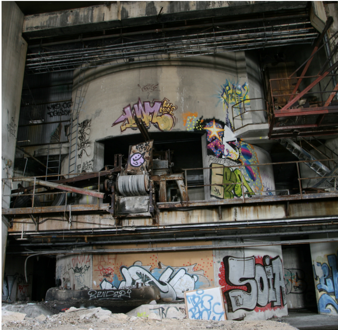
Figure 28. View towards silo 2, a balcony of concrete runs in front of the silos at the 1st floor. The openings in the front are about 4x7 meters.
