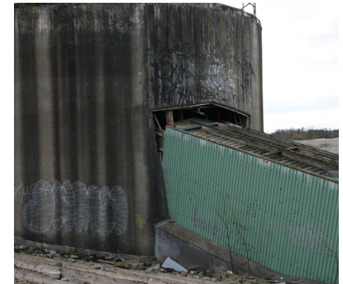
Figure 35. Existing opening towards west.
