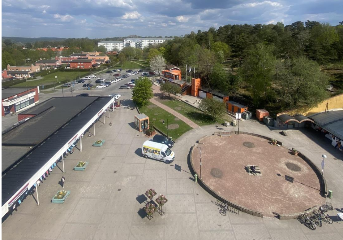
Figure 4.8 Hammarkulletorget with premises for different operations to the left, the container building Mixköket in the middle, and the tram stop to the right.
