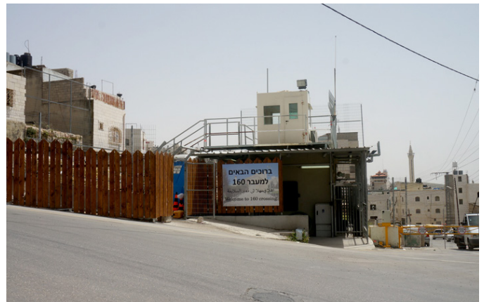
D. 160 Checkpoint separating H2 Area from the southern neighborhood in H1 Area. Source: Eyal Hareuveni, B'tselem.
