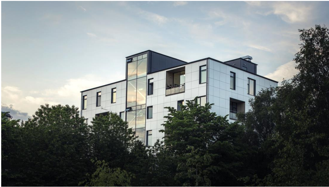
Figure 2 HSB Living Lab Building
