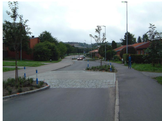
Figure 4.3: Side moved road, here with a speed bump. Photo: Vägverket Region Mälardalen
