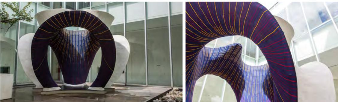
**Figure 2.3:** KnitCandela pavilion with the textile framework kept in place [8]
