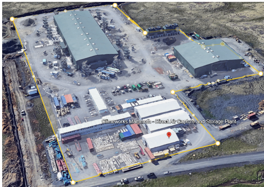
Figure A.2: Satellite view of the Climeworks Mammoth facility.
