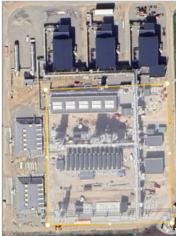
Figure A.6: Combined footprint of the methanol synthesis and compressor units. Author's own measurement via Google Earth, 2026
