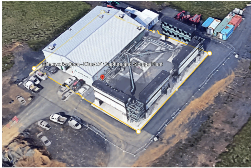
Figure A.1: Satellite view of the Climeworks Orca facility.
