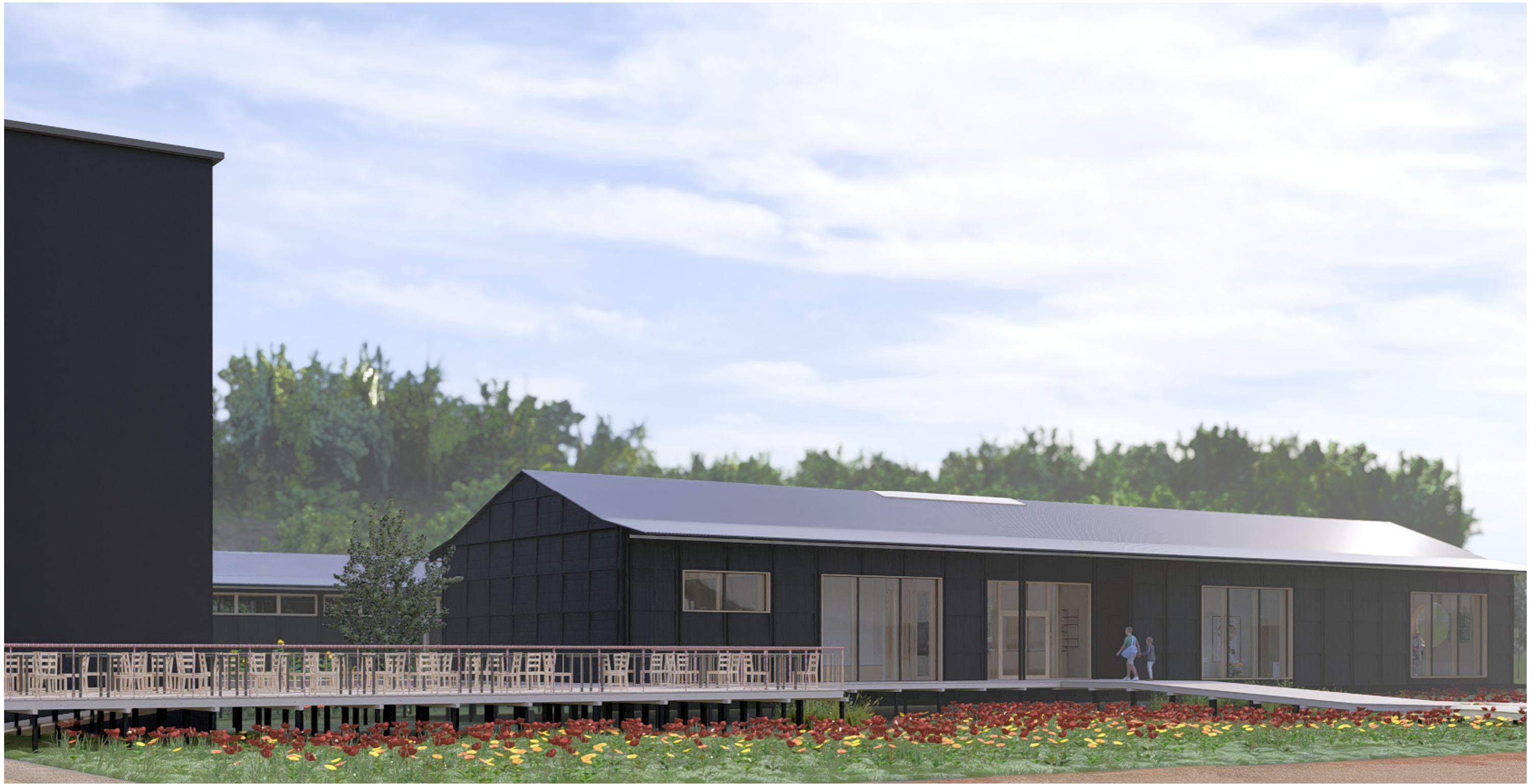
Approaching the site.
