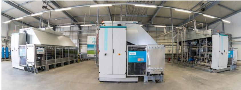
Figure 4.9: High pressure, 3.5 kA stacks as installed in Energiepark Mainz in Germany [39].
