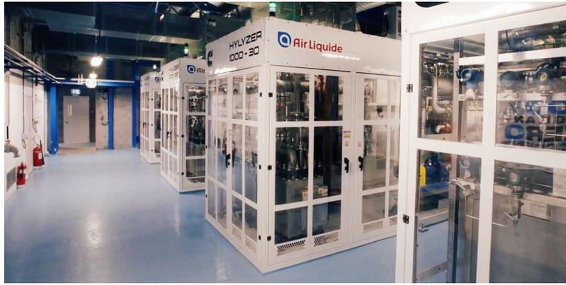
Figure 4.10: Based around a modular 20 MW PEM electrolyser, the new facility in Canada doubles Cummins previous installation size in Japan [47].
