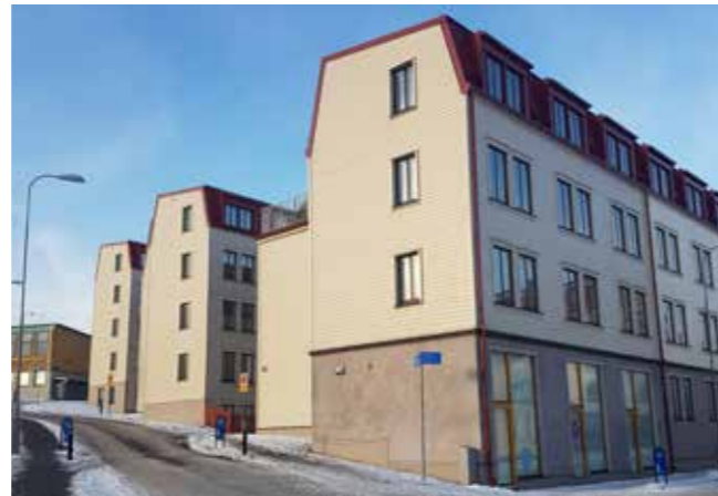
Photo: Plejadgatan is a good example of how Light Frame Volumes can be completed with a site built facade to fit into the cityscape
