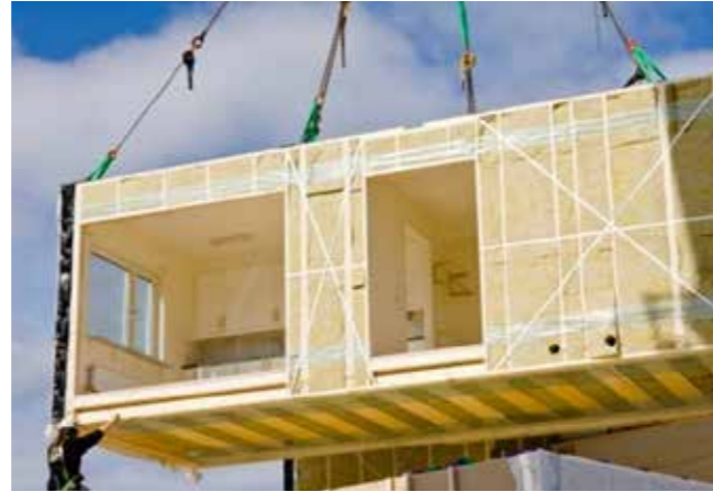
Figure 33. Light Frame structures are usually prefabricated as Volume Elements and swiftly assembled at site. (Affärer i Norr, 2017)
