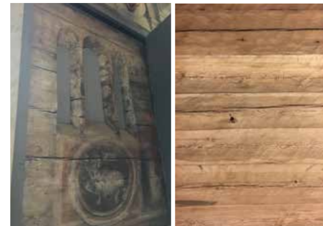
Left: Original window from the mid 13th century from a time when glass was a rare commodity. Therefore small openings with filleted edges were made to let more natural light in. Right Marks from the crafts-persons tool.
