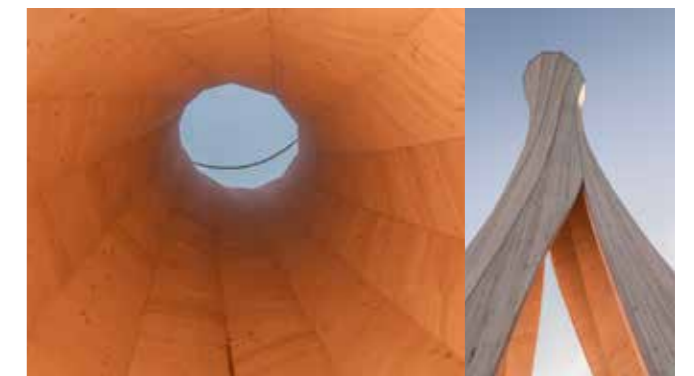
Figure 31. The research project Urbach Tower is an example of how the Surface Active behavior of CLT opens up a range of new structural possibilities with wood. (ICD/ITKE, 2019)
