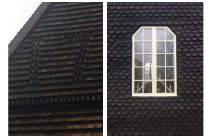
Left: Playful ornate facade showing the year of a large renovation Right: Wooden shingles around window of the church facade.
