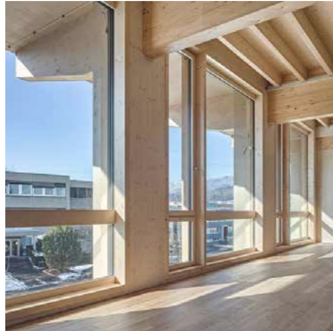
Figure 27. Since all loads are transferred in the Posts/Columns the spaces in between can be left open. (Baunetz, 2017)
