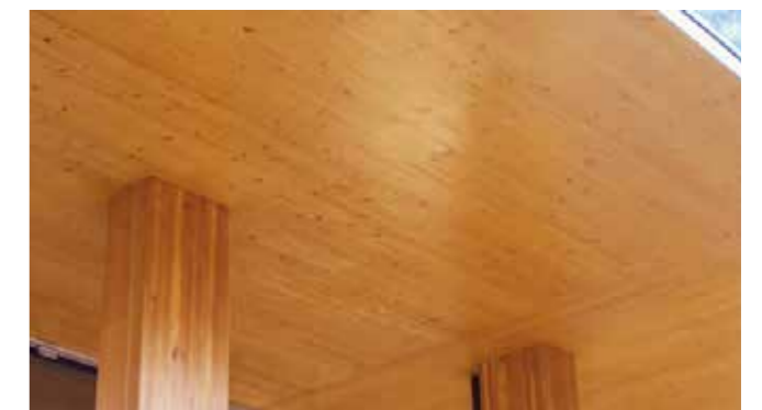
Figure 32. Because of the ability to redistribute forces a CLT-slab can be single supported on top of a pillar without a supporting beam. (Apawood, n.d.)
