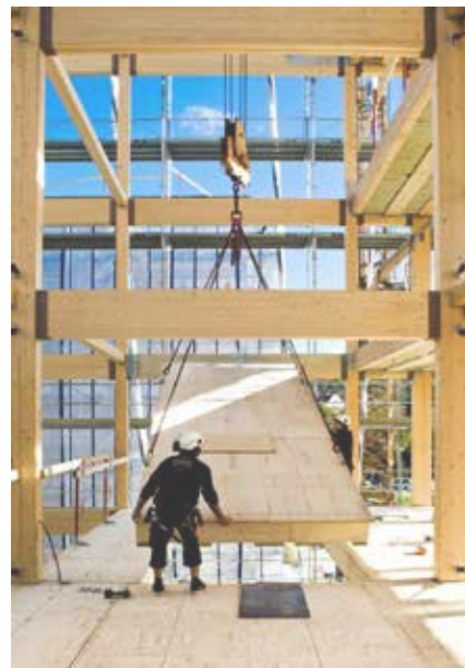
Figure 24. Post-Beam - Housing Project (Moelven, 2012)
