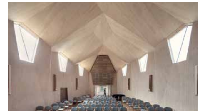
Figure 30. The chapel from Nicolas Pople Architects is a great example of how CLT-slabs can form a folded plate structure with a large span without beams or pillars. (Dezeen, 2020)
