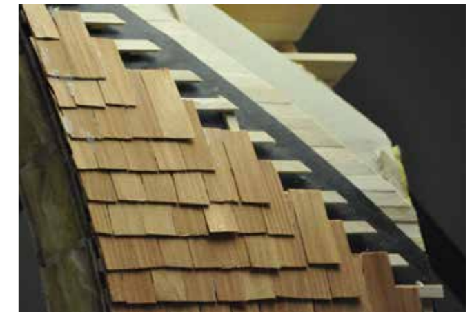
Glulam arch with shingle panel
