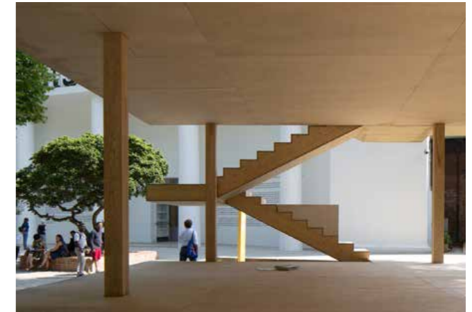
Figure 11. Le Corbusier’s seminal Maison Dom-ino entirely made out of wood (Fearson, A. 2017)
