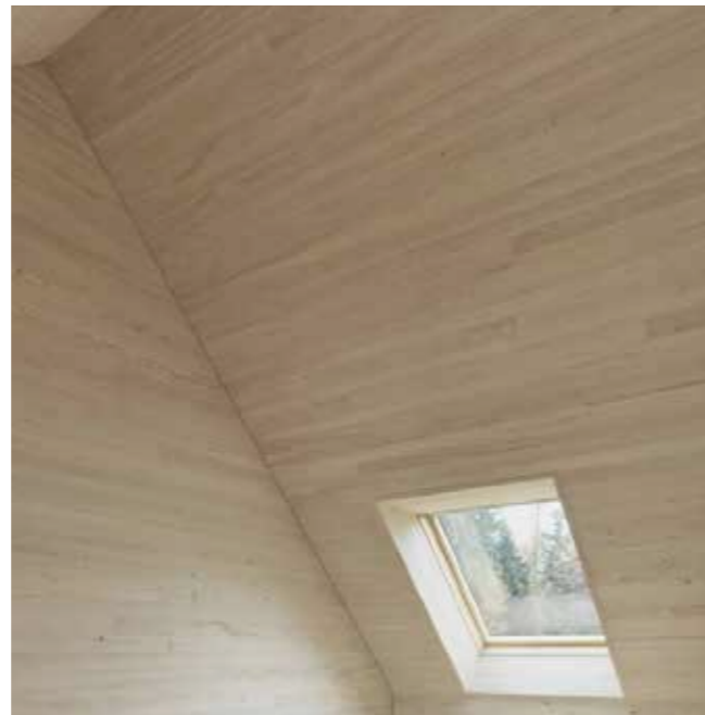
Figure 5. Airtightness makes the CLT construction perform well as a low energy and passive house (Von Radina, 2014)
