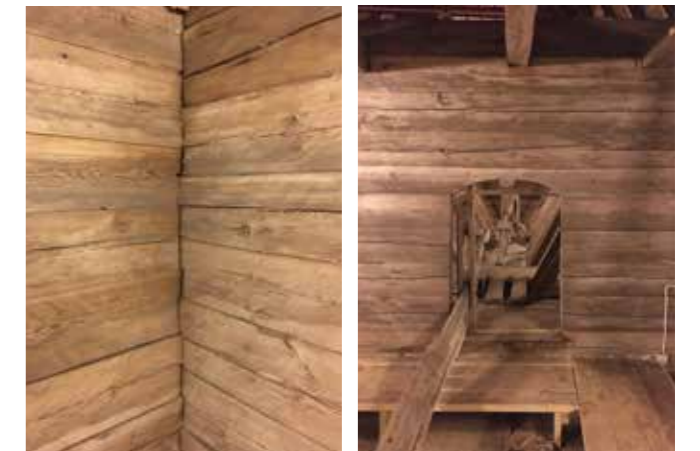
Joints and interior apertures in the solid wood made entirely without screws and / or nails.
