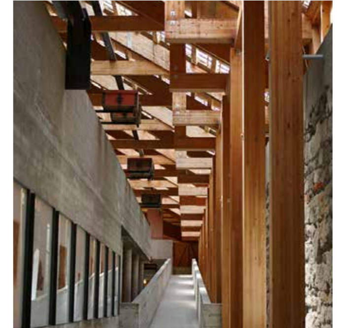
Figure 22. Hedmark Museum Sverre Fehn uses materials and geometry of the structure to tell his architectural story (Peter Guthrie, 2013)
