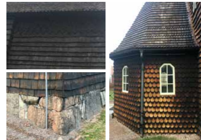
Left: Accentuated plinth and soffit. Right: Patina of facade depending on how exposed the surface is.
