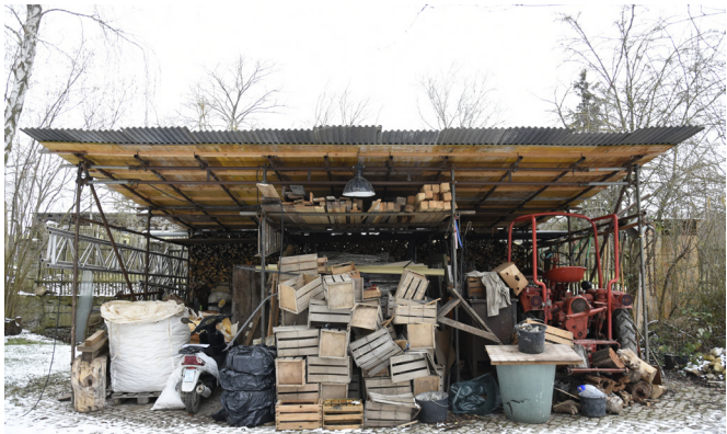
Figure 28 The equipment shelter February 2025
