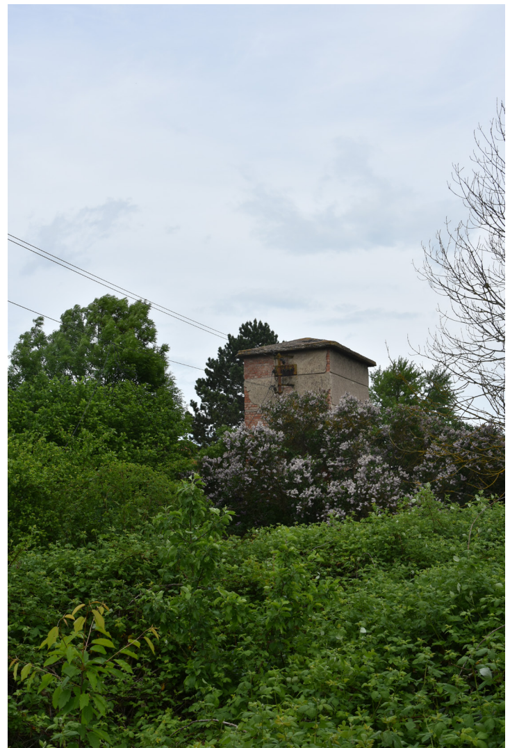
Figure 16 Flora in front of the substation May 2022
