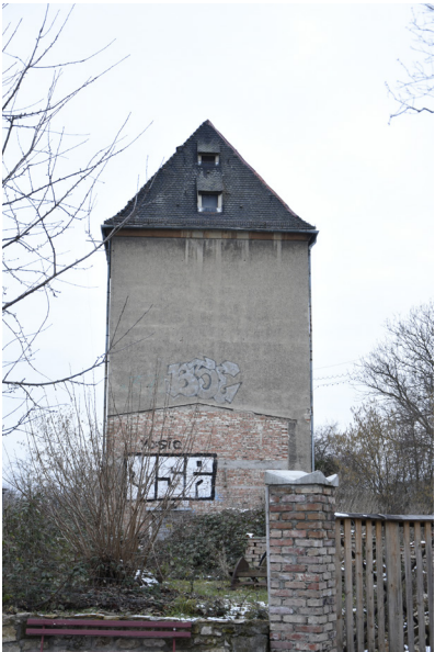
Figure 22 The silo February 2025
