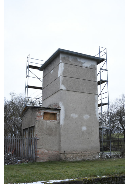
Figure 25 The substation February 2025
