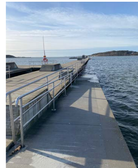
Figure 43: Photo of ramp.
