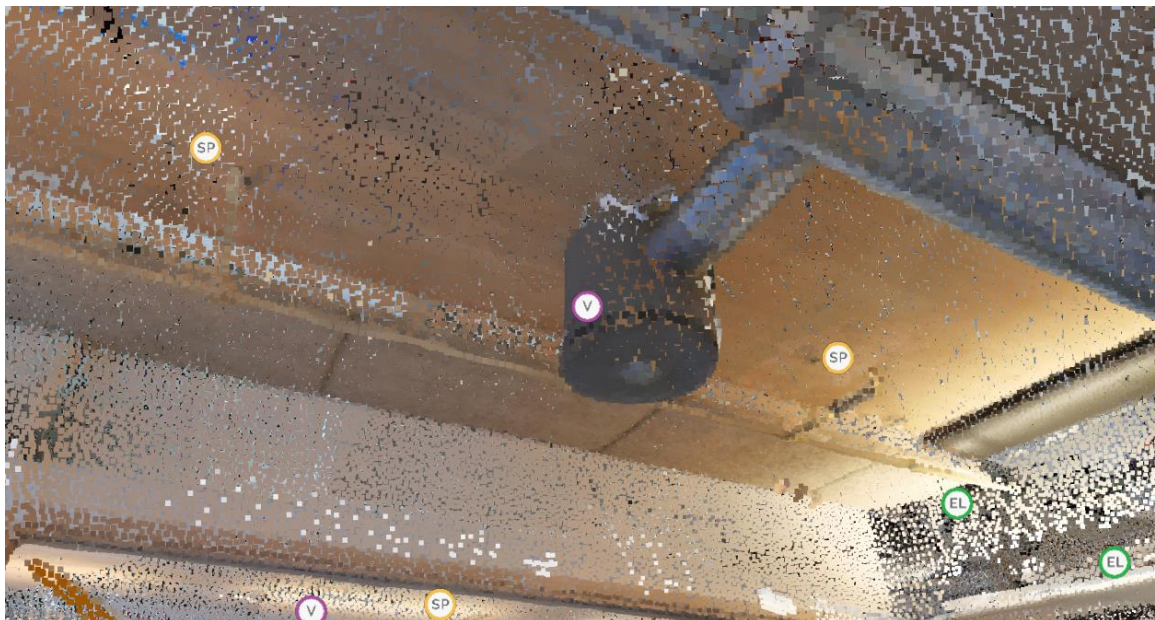
Figure 6 Point-Cloud screenshot containing HVAC system in the ceiling. (Zynka BIM, 2021)
