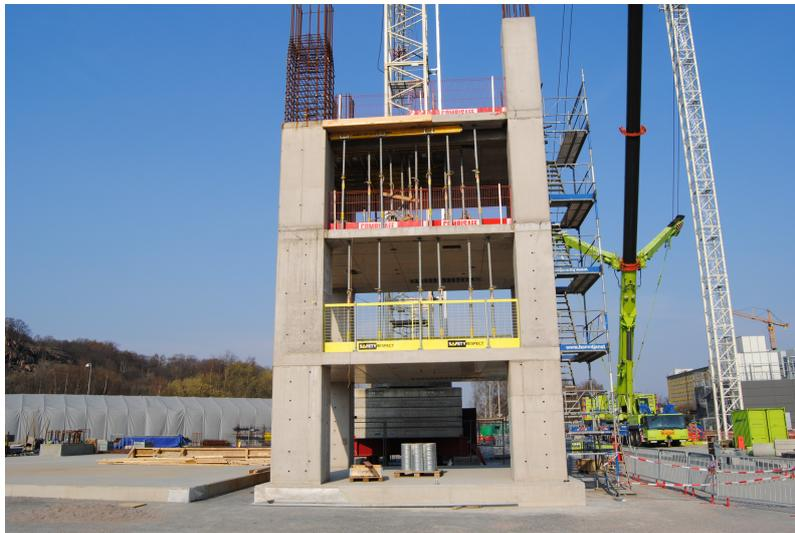
**Figure 2.3:** *Backpropping in one multiple floors.*
