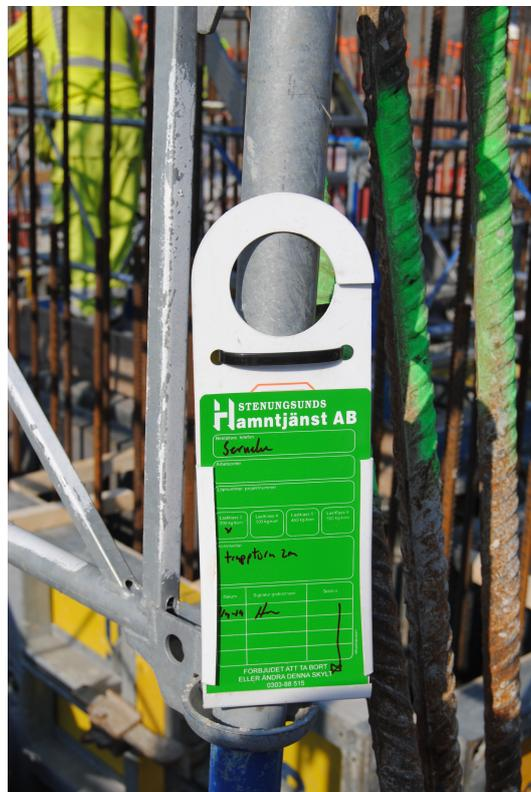
**Figure 2.7:** *An example of a sign which display's an approved inspection of the scaffolding on the entrance of the scaffolding.*
