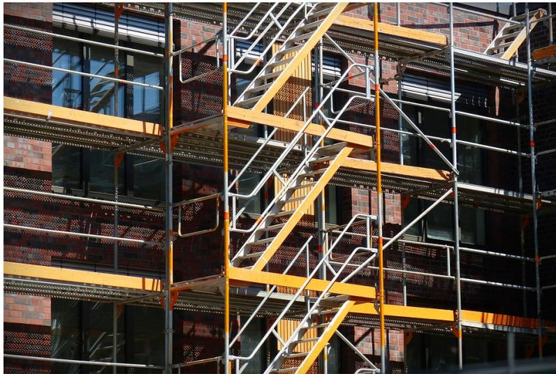
**Figure 2.6:** *An example of scaffolding providing working space along the façade (Bernswaelz, 2016).*
