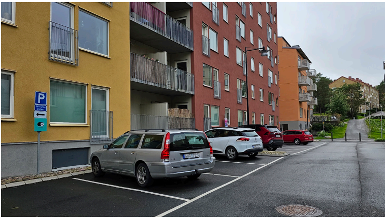
Figure 21a. Residential block with parking spaces just outside the apartments. Not an optimal solution as the lights from the cars will light up the apartments, in addition to the noise from the cars. Large windows allows for much daylight, but will also have privacy issues on the ground floor.
