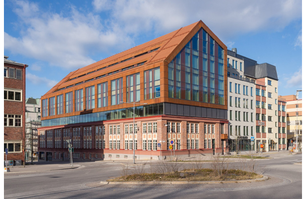
Figure 28a: Exterior of Trikaafabriken, showing the original brick building and the roof-top extension. Picture by Arild Vågen / Wikimedia commons CC BY-SA 4.0,
