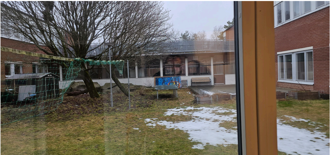
Figure 35a. Picture of the former youth center, Tyrolen. It is not used due to a mold infection in the ceiling.
