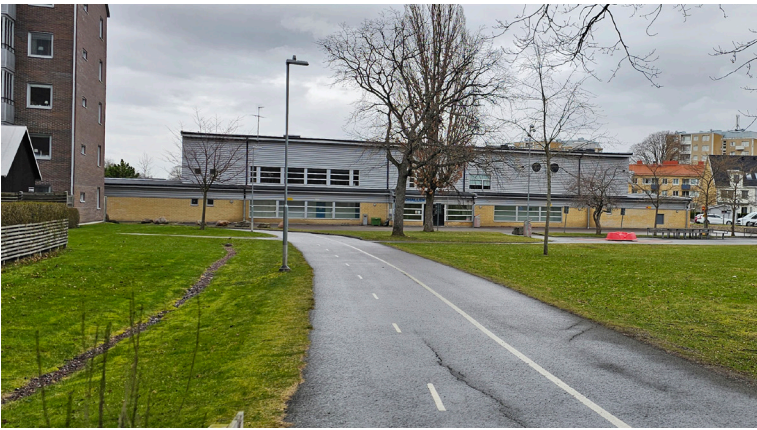
Figure 18b. Heidhallen, the only remaining structure from Jämbrottsskolan. The space in front of the building is an open space with no clear function, just some pavement and a grass lawn. It seems unclear, uninviting and unattractive.
