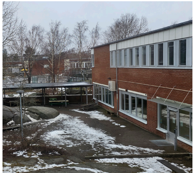
Figure 34a: Red brick facade, white lintels and continuous ribbon windows. The windows on the ground floor were changed in 2021 and the ones on the first floor were changed in the 1980's.
