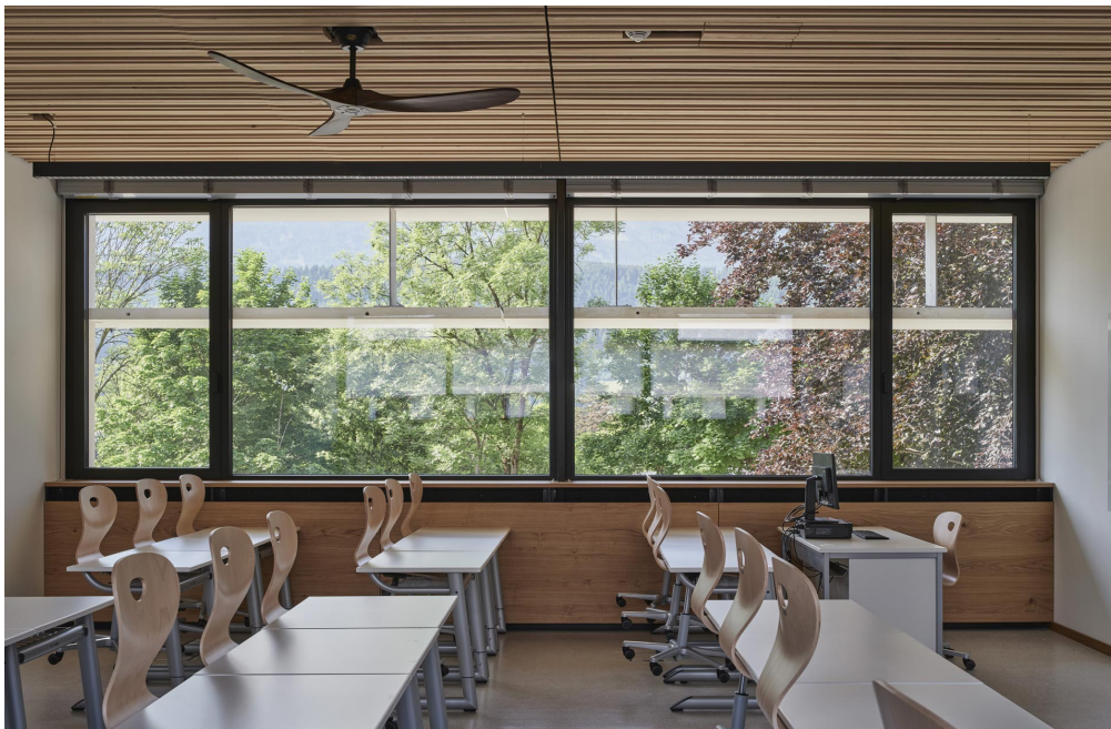
Figure 29b: Picture showing the classroom. The wooden box below the windows is where the trickle-vent is located. The fan on the ceiling further enhances the air quality during the warm summer days. Picture: Günter Richard Wett
