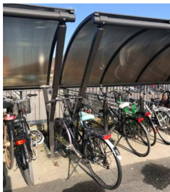
Figure 55. Unwanted gap between two sections
