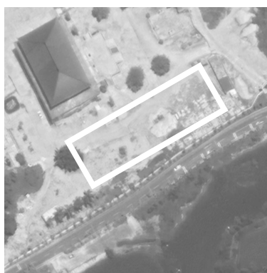
4. Guangfu Temple Parking lot (under construction)
