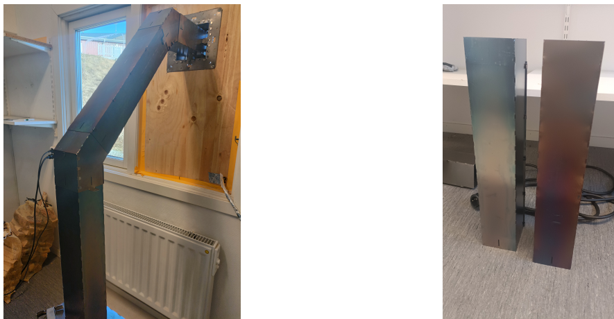
Figure 5.7: Chimney installation and components: The left shows the stove with the chimney mounted to the window board, and the right shows the chimney components.
