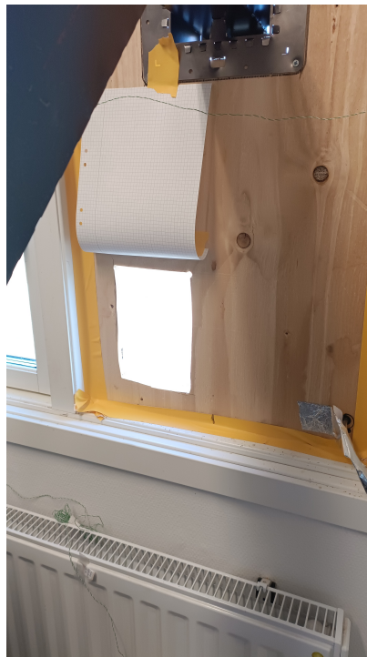
Figure 5.16: Opening on the window board below the chimney
