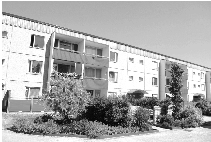
Figure 3.3 Case study building before renovation.
