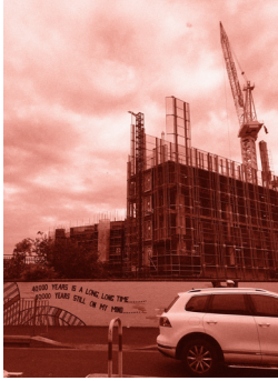
THE BLOCK, REDFERN SITE VISIT
