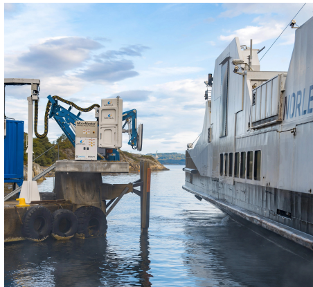
Figure 1.5: The electrical ferry "MF Folgefonn" with stationary IPT system in Norway
