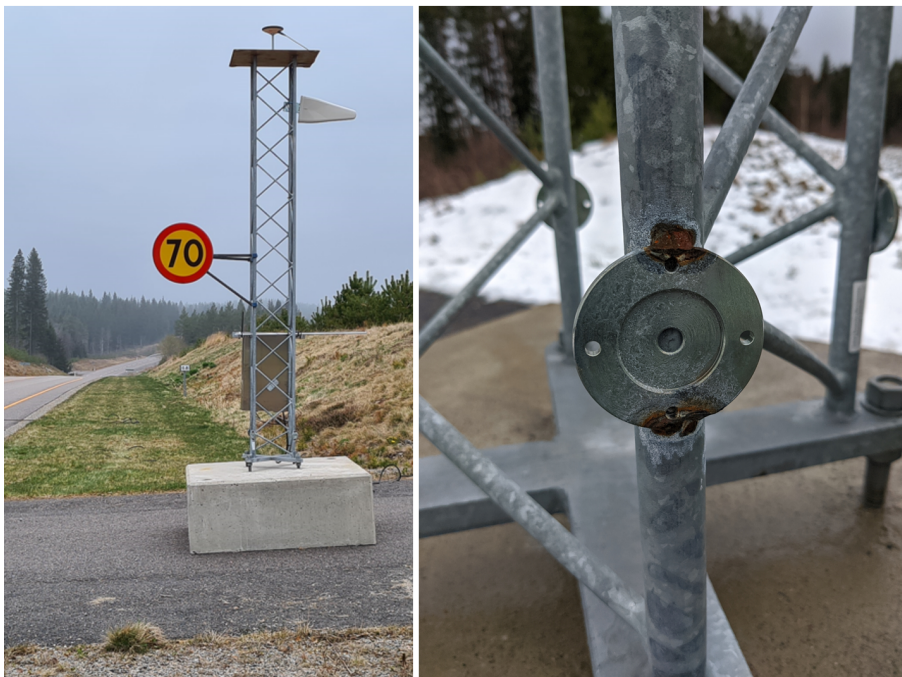
Figure 3.2: Truss mast standing on ground with speed limit sign mounted (left) and mounts for the magnetic ball base to place reflecting prisms for laser scanner measurements(right).
