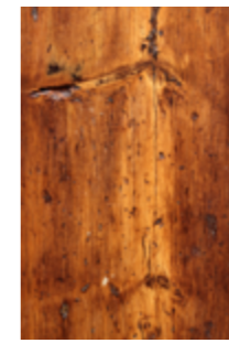
Facade wood panel
