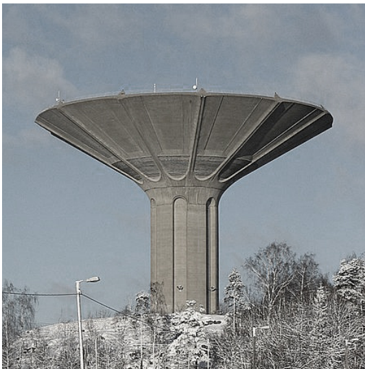
The mushroom tower in Helsinki. Picture: Water tower Helsinki Finland. (n.d) Retrieved 31 mars from Wikimedia, https://commons.wikimedia.org/wiki/File:Roihuvuori_water_tower_-_Helsinki_Finland.jpg
