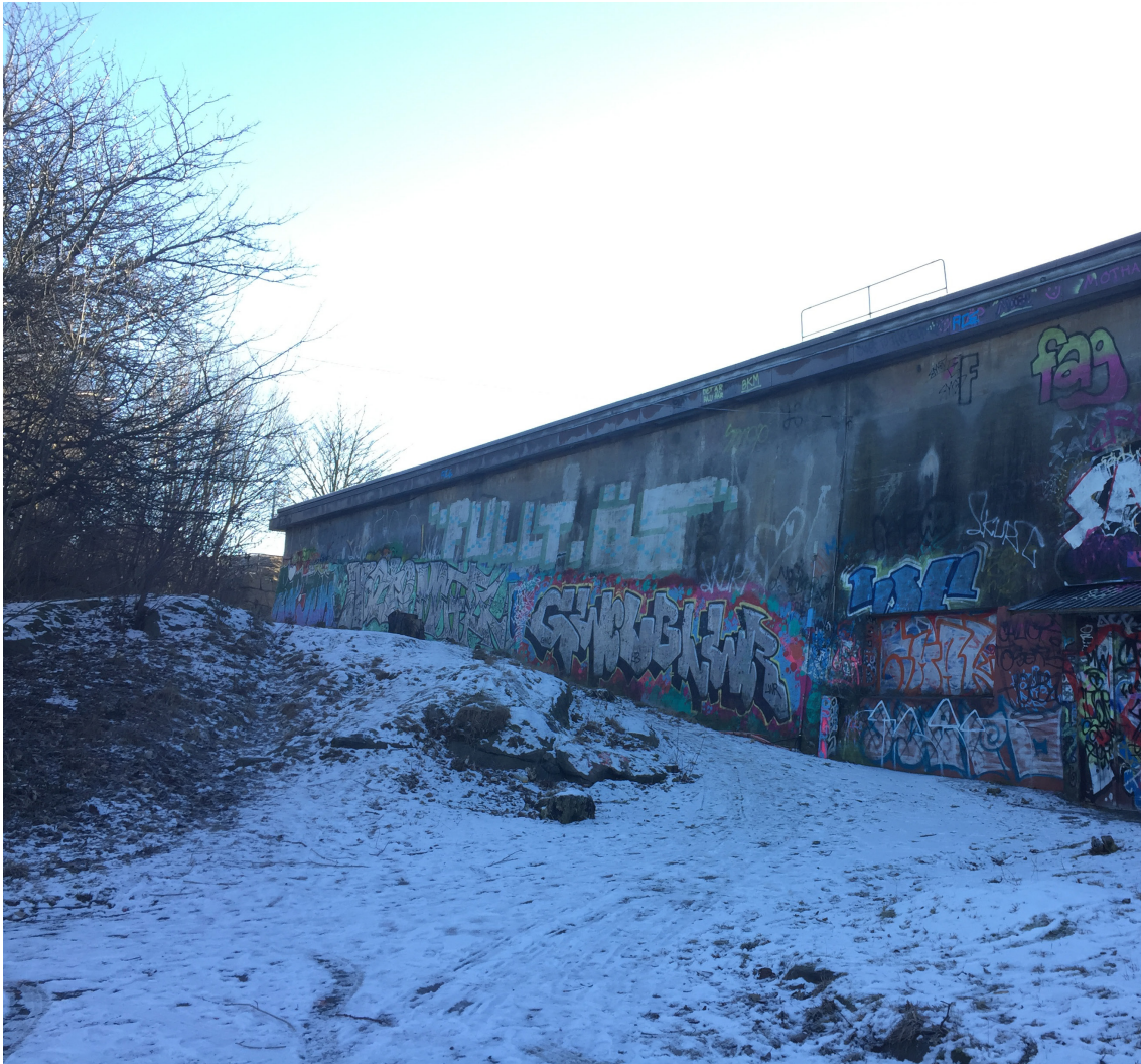
The new reservoir is still in use and is situated right next to the old one. Picture: Ellen Linder
