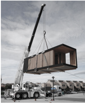
Figure 49 - 50: Prefabricated CLT modules/ Urban design concept – 50 Modular Timber Apartments. Note: Reprinted from Philippe Ruault (n.d.) via Pinterest and ArchDaily.
