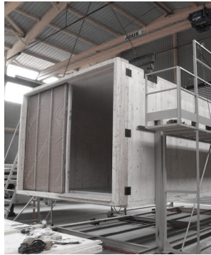
Figure 49 - 50: Prefabricated CLT modules/ Urban design concept – 50 Modular Timber Apartments. Note: Reprinted from Philippe Ruault (n.d.) via Pinterest and ArchDaily.
