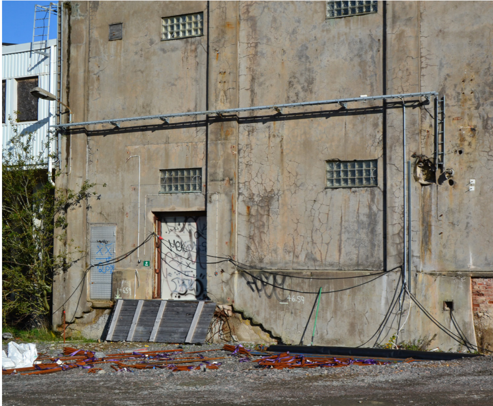
Current condition of the southern facade.
