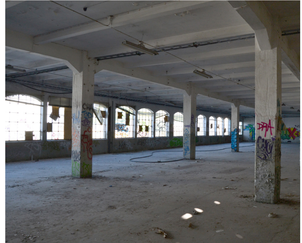
The interior with its concrete column structure.
