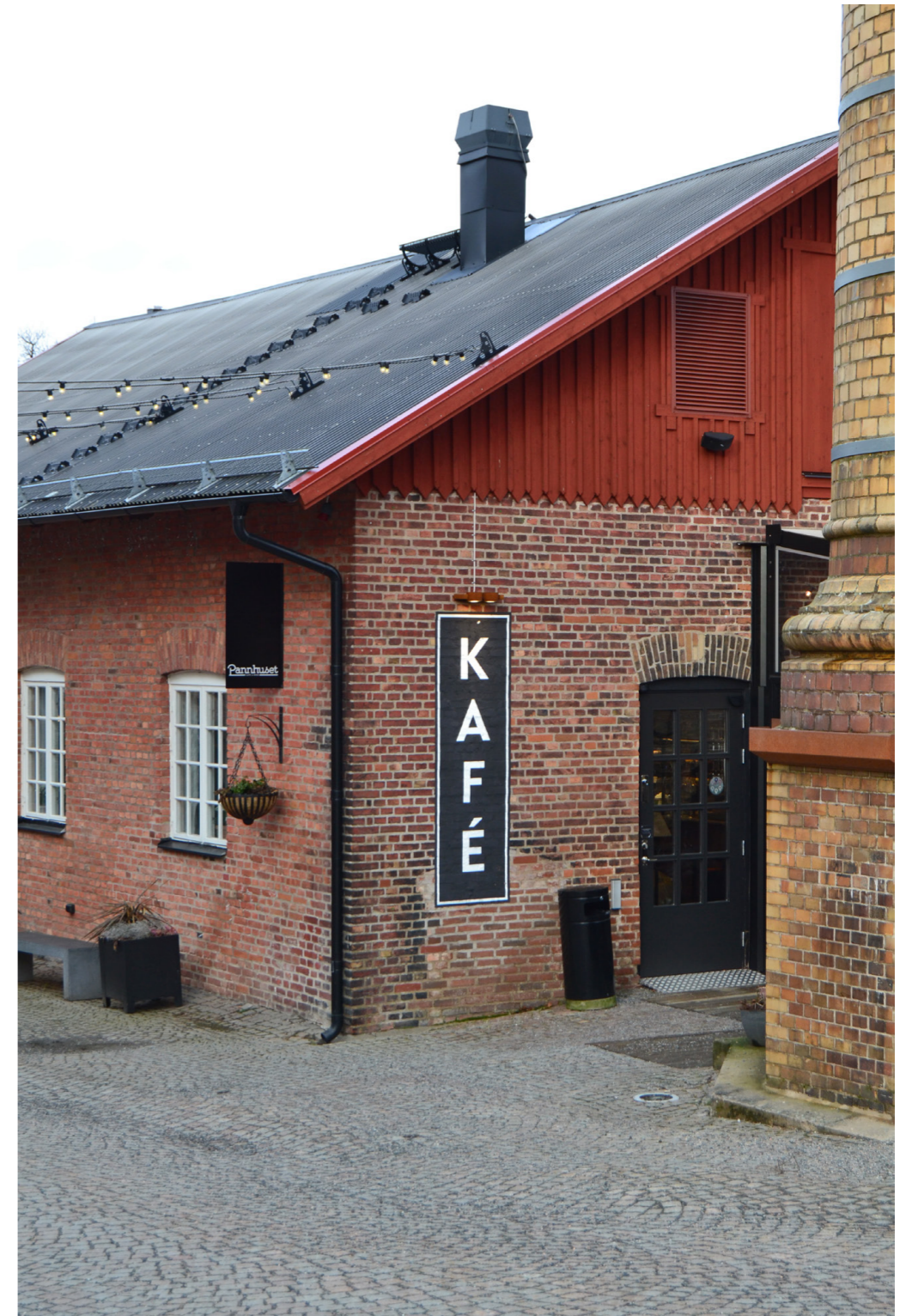
Factory building converted into a café at Nääs Fabriker
