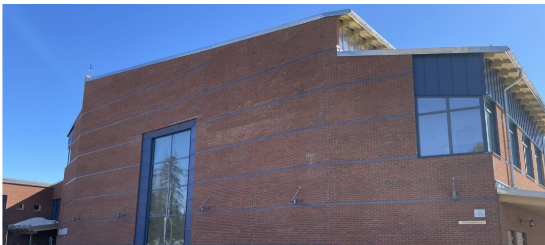
Figure 5: Part of the building in project B which was not demolished, to show the characteristics, Photo: Per Hilmersson (Akademiska Hus), personal communication, 2026
