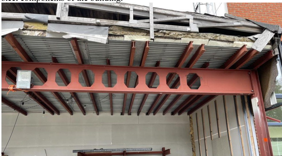
Figure 6: The demolition process of project B, showcasing the steel elements, photo: Per Hilmersson (Akademiska Hus), personal communication, 2026
