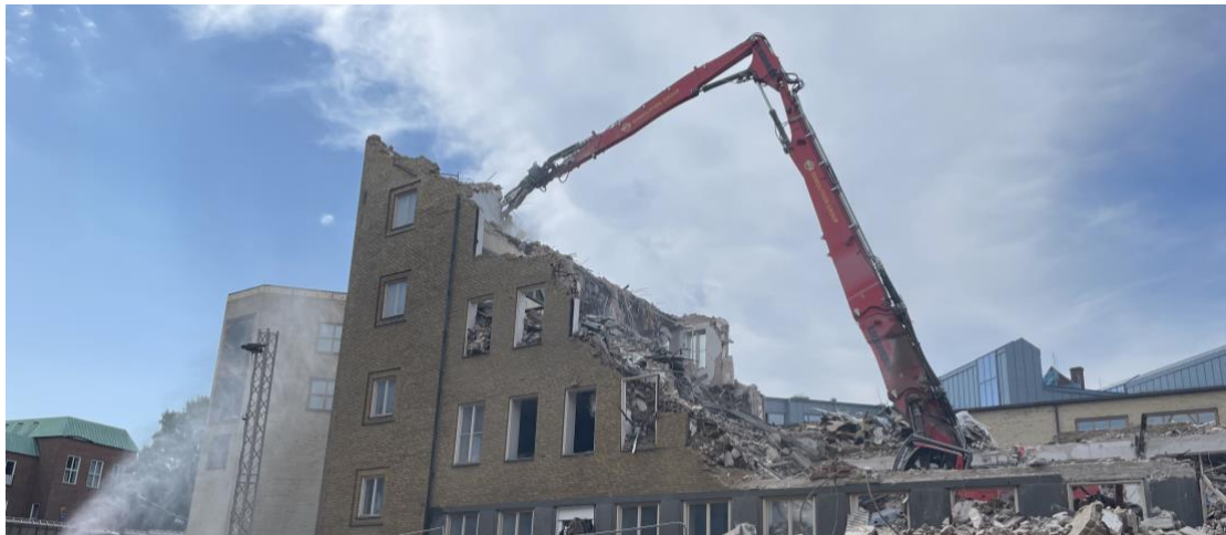
Figure 4: Demolition of main building in project A, Photo: Per Hilmersson (Akademiska Hus), personal communication, 2026
