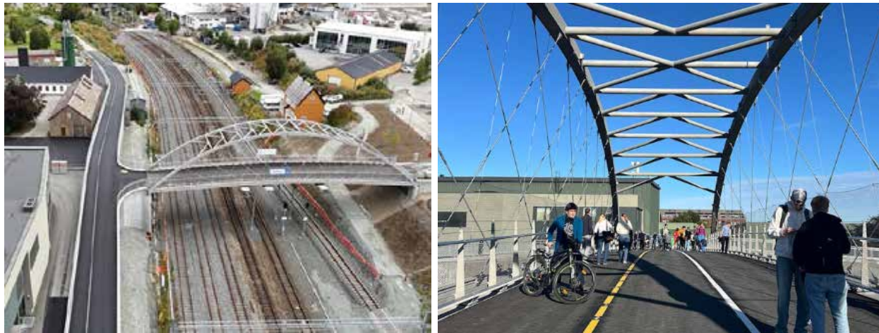
Figure A : Hangarbrua going across the railroad tracks at Leangen station in Trondheim, Norway. (Photo credits: Vegard Thorvaldsen/Statens vegvesen)
