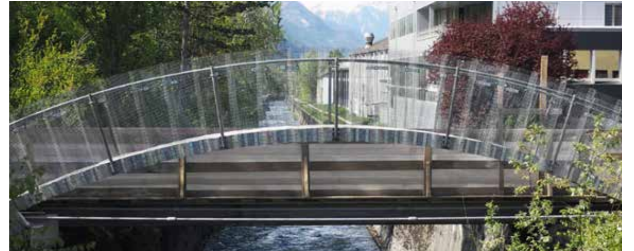
Figure B: The Re:Crete footbridge
