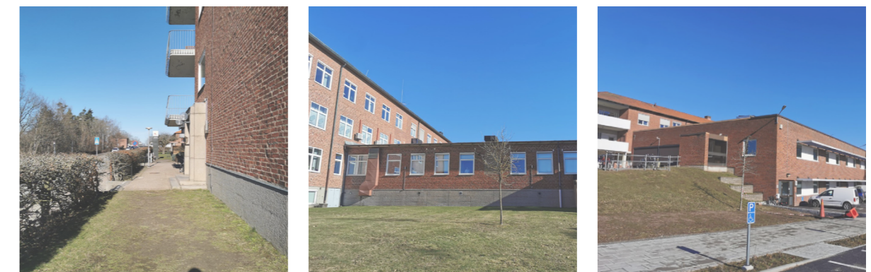
Green barrier beside the public road
