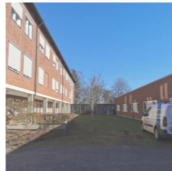
Extension building pathway (site)
