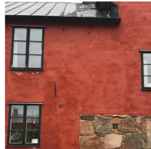
Render, stone & metal sheet roof
