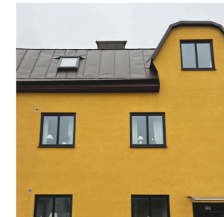
Render & metal sheet roof
