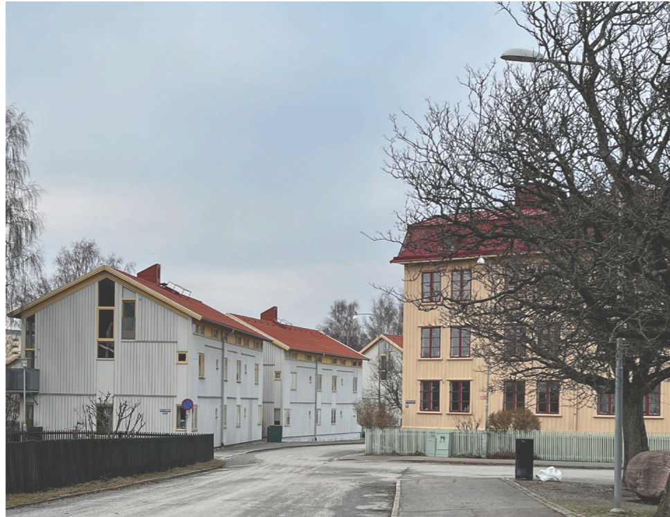
Photograph of Gamla Lindholmen, new buildings on the left and older house to the right.
